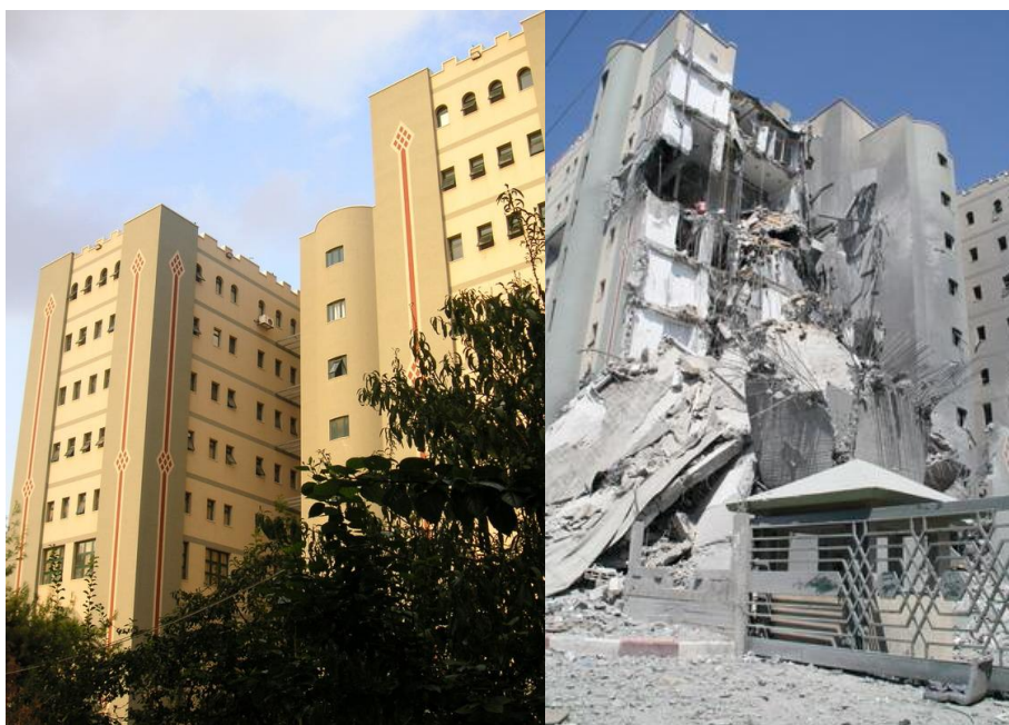
Ministry of Planning before destruction
